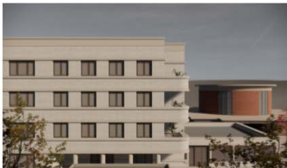
Banding to head & sill - Homogeneous with light brick
